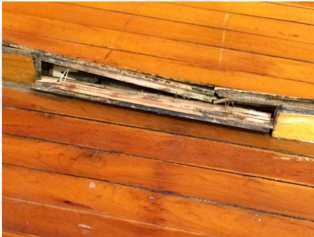
Repair Buckled Floor Boards
