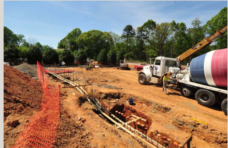
Wall Footing Excavation with Reinforcement
