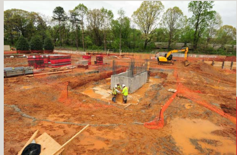
Foundation and Pit at Elevator Hoistway
