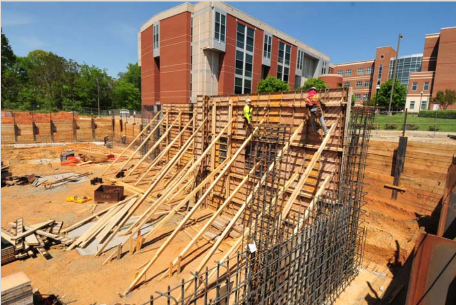
Erecting Formwork for Retaining Wall
