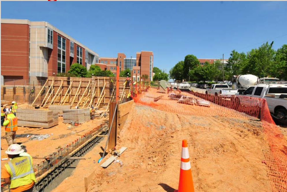
Site Looking East Towards WB Atkinson and Computer Science
