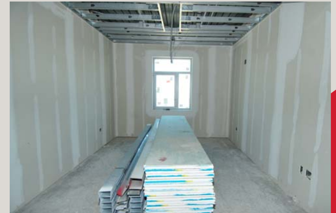
Typical Bedroom with Drywall Application
