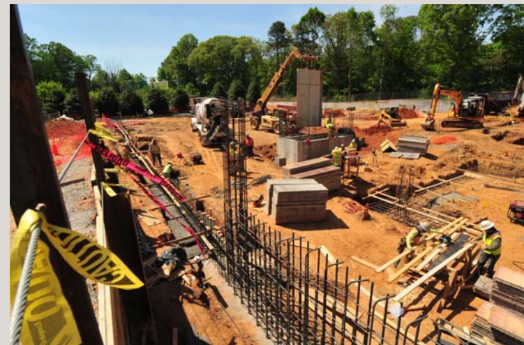
Erecting Formwork for Elevator Shafts
