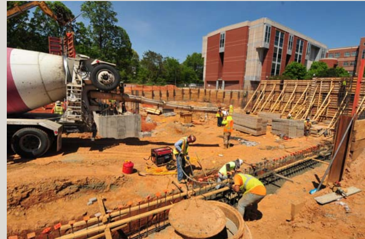
Pouring Footings for Foundation Wall
