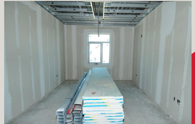
Typical Bedroom with Drywall Application
