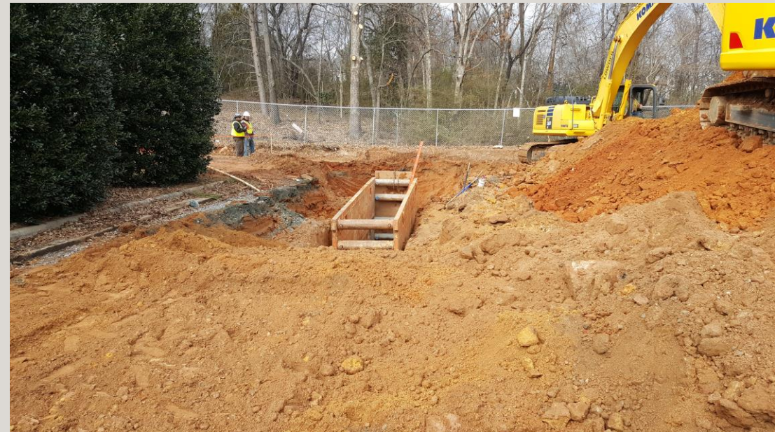
Trench Box to prevent cave-ins while laying pipes
