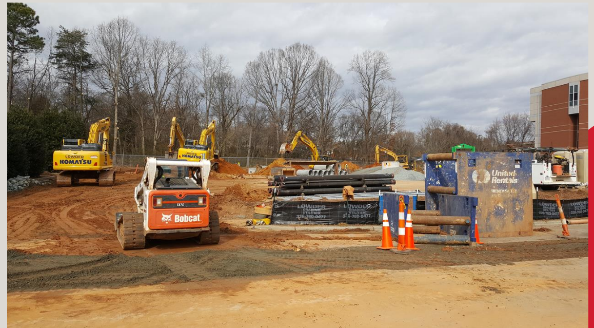
Construction Site looking north w/ WB Atkinson to right
