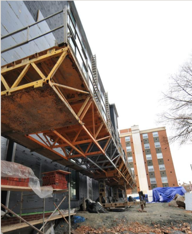
Exterior Masonry Installation
