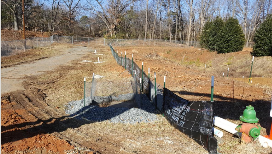
Temporary access road at west side of site
