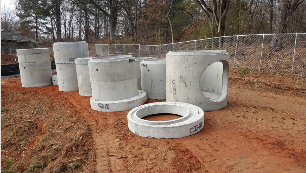
Prefabricated Storm Drainage Manhole Sections
