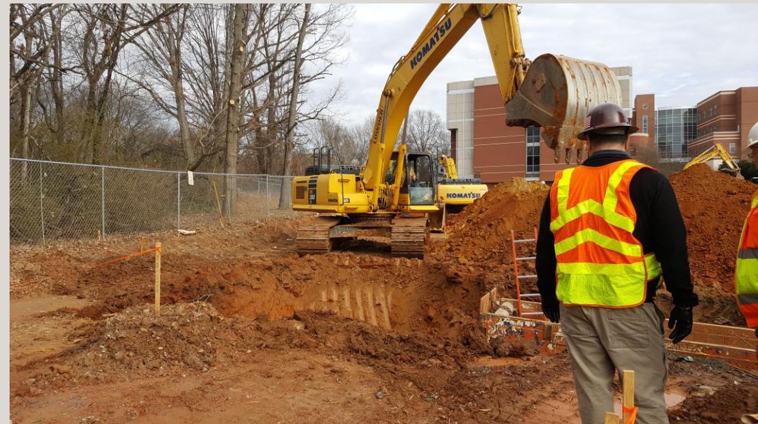
Excavator prepping trench to install Manhole
